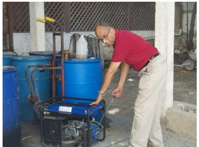
Jean-Robert, HH2JR, struggled to keep the generator working throughout the contest at 4V1JR. [Dale Long, N3BNA, photo]
