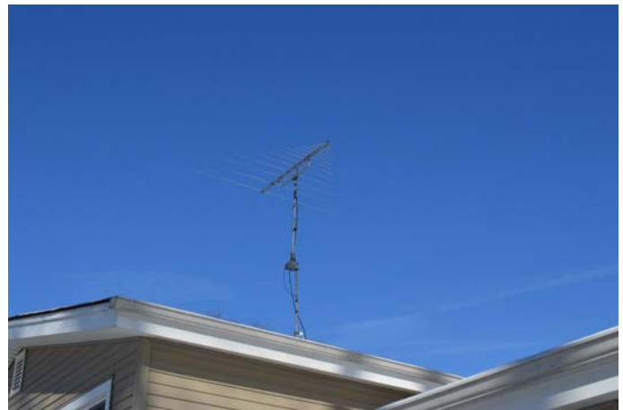
KO9A's log-periodic array. (KO9A photo)
