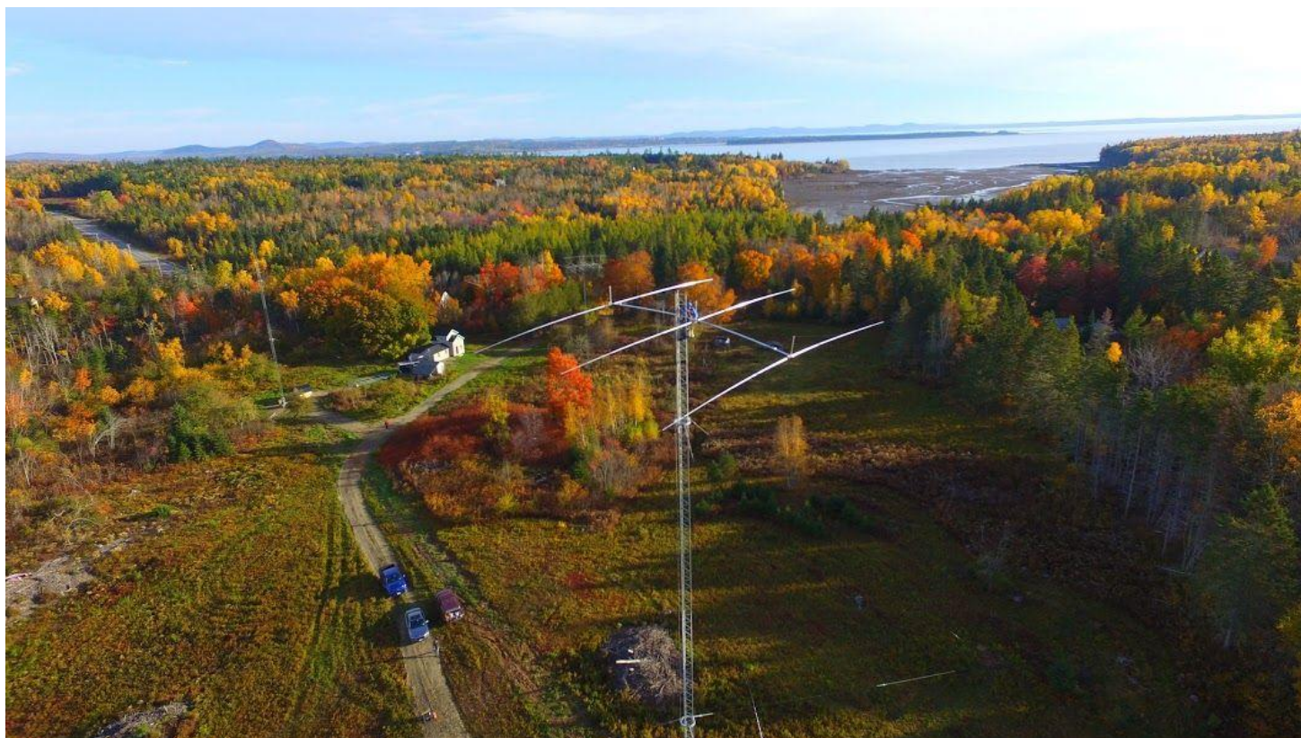
40-meter beam at the Eastport, Maine remote station... saltwater, saltwater. (Photo – Ray Higgins, W2RE)
