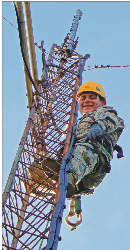
Figure 1 — Cadet John Humelsine, WA4BUD, smiles from our repeater tower before he proceeds to install a new 2-meter antenna. [Matthew Sherburne, KF4WZB, photo]
